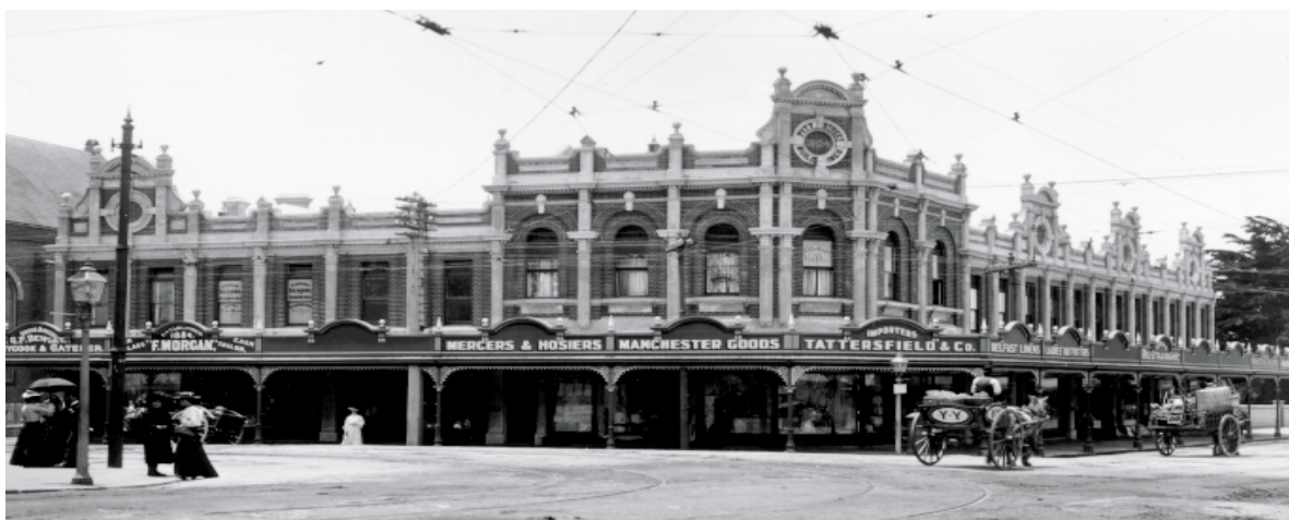
Pitt Street Building, December 1904
