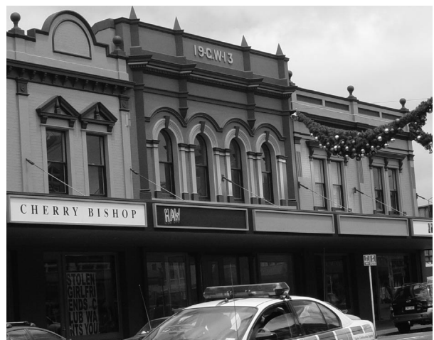
Modern verandahs hung from the building by tension stays create an open-sided space
