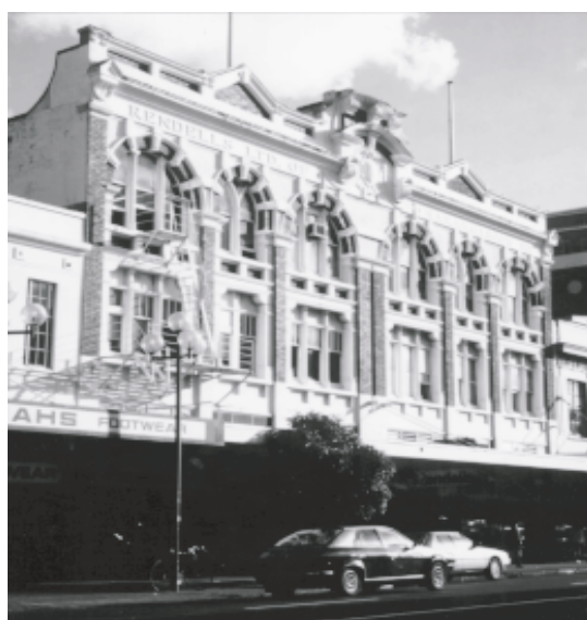
A plaster frontage with brick trim around window openings, in spandrel panels and at parapet level
