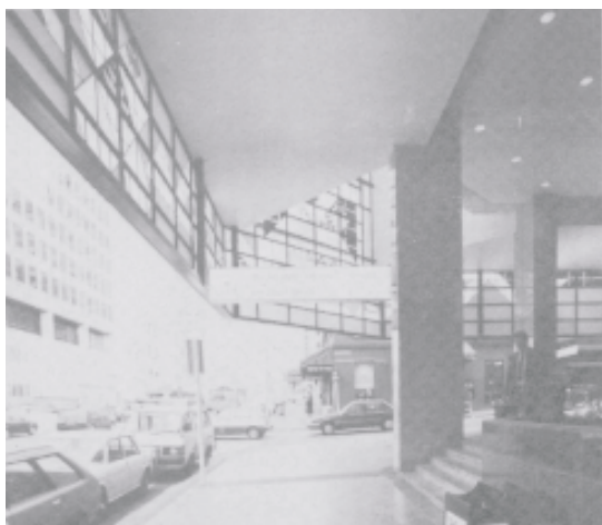
Cantilevered curved verandahs (or high flat verandahs with “shelter skirts” dropping from the outer edge) maintain a sense of containment
