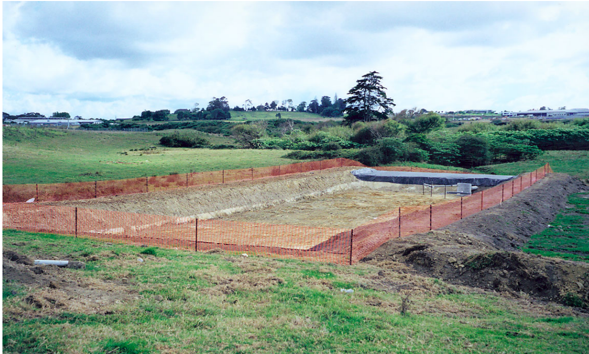
Photo 7.8 Sediment Retention Pond
