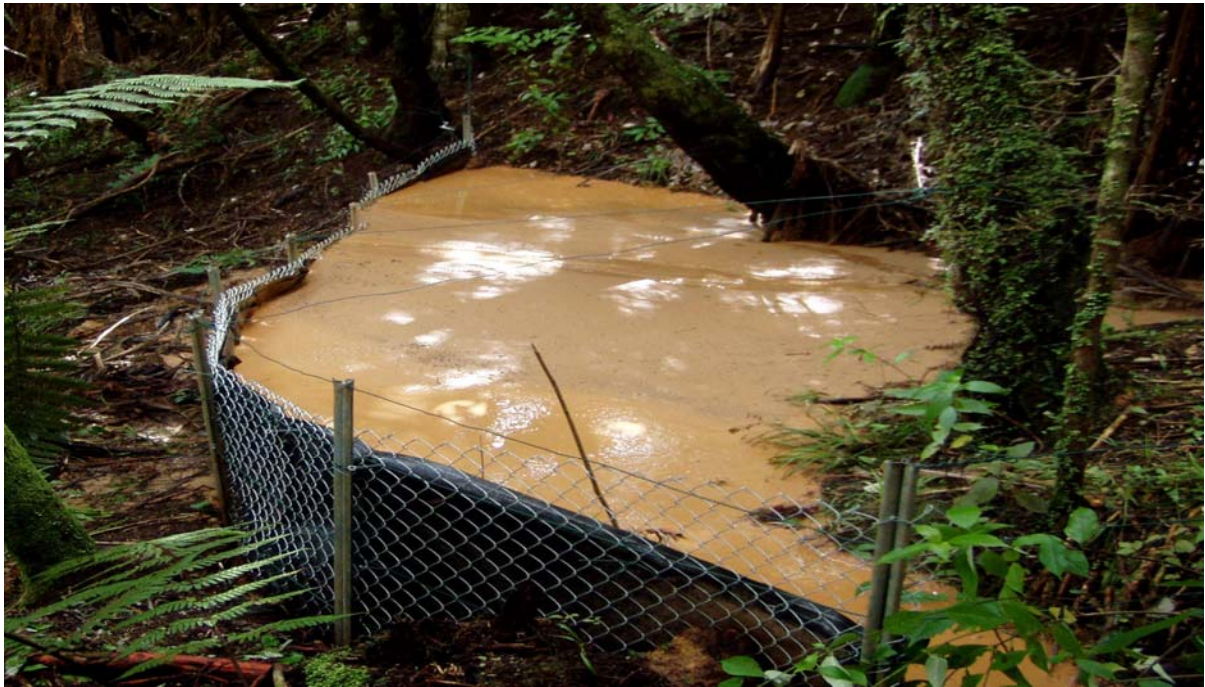
Photo 7.3 Super silt fence used as a debris dam to contain mobilised sediment
