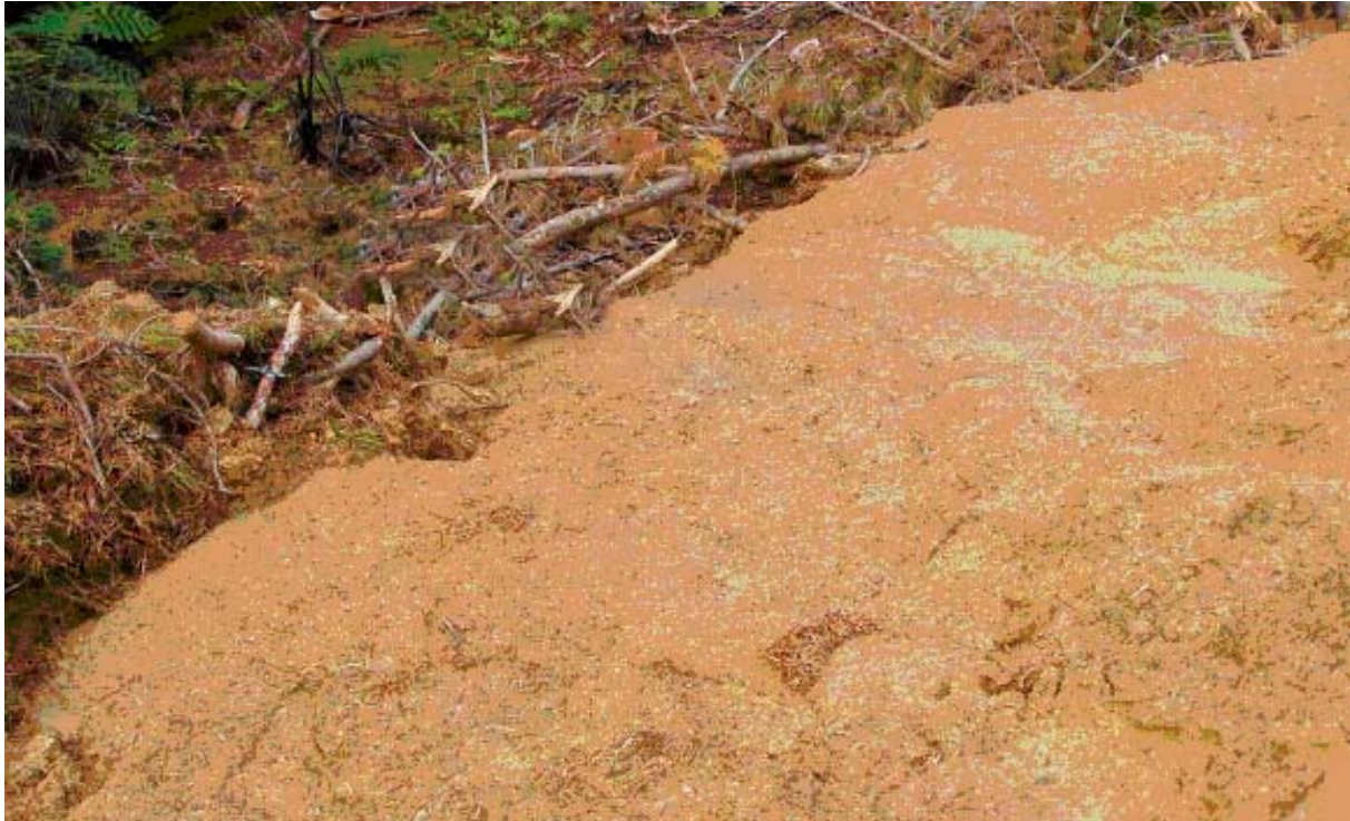
Photo 7.4 Example of slash bund used to impede the flow of a sediment 'slug'
