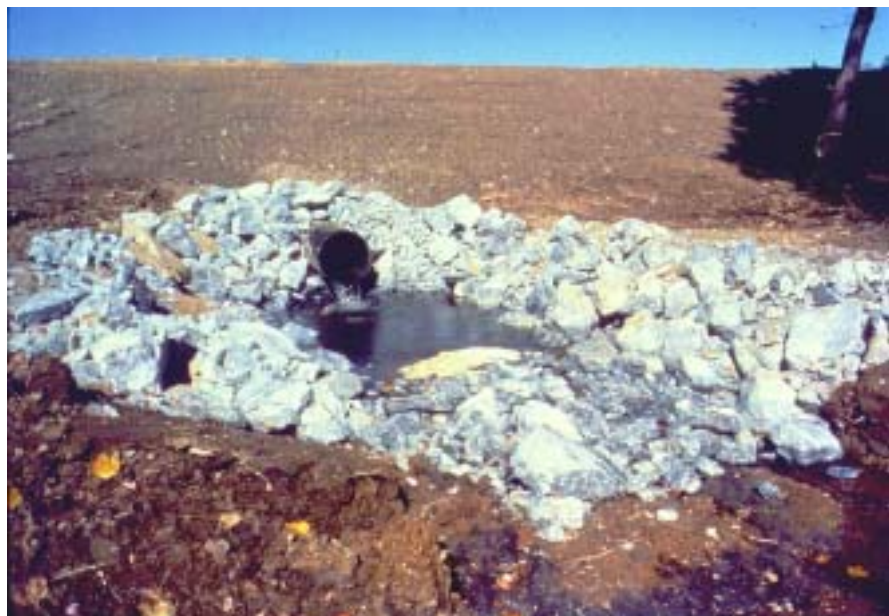
Plate 13-1: Example of riprap at a stormwater outfall
