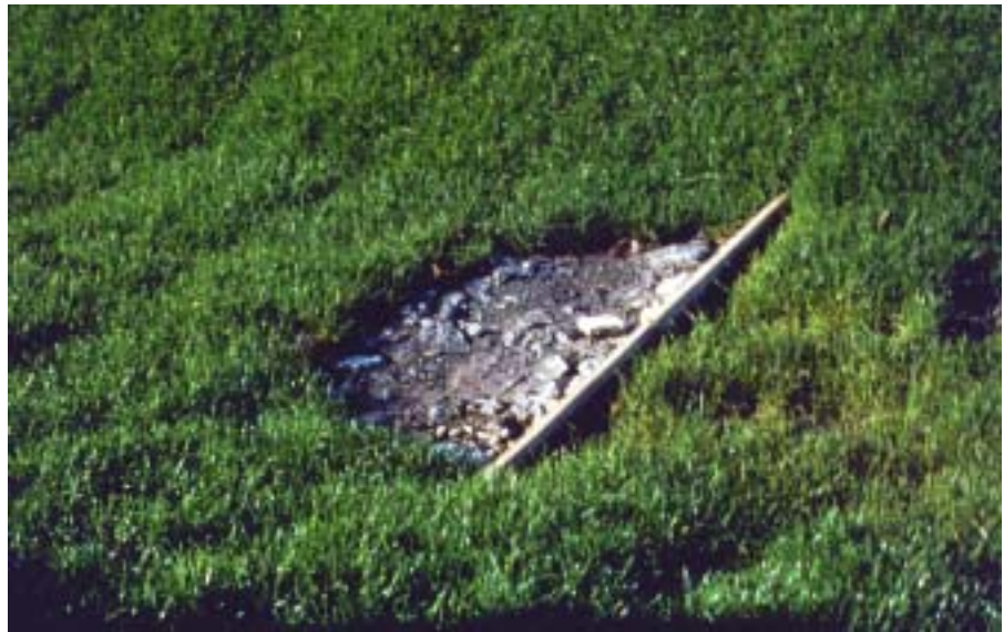
Plate 9-3: Detail of a swale check dam
