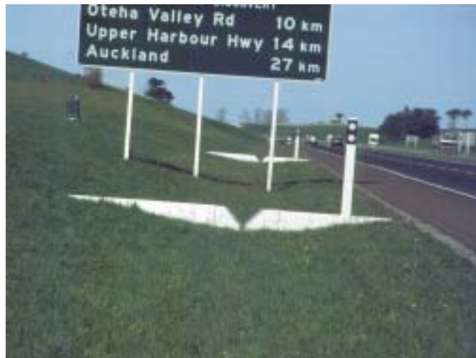
Plate 9-2: Swale monitoring location south of Silverdale
