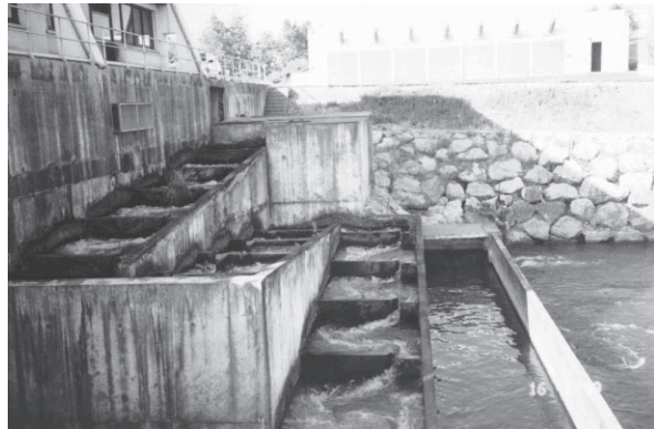
Plate 21: Vertical slot fishway retrofitted to a small power plant.
