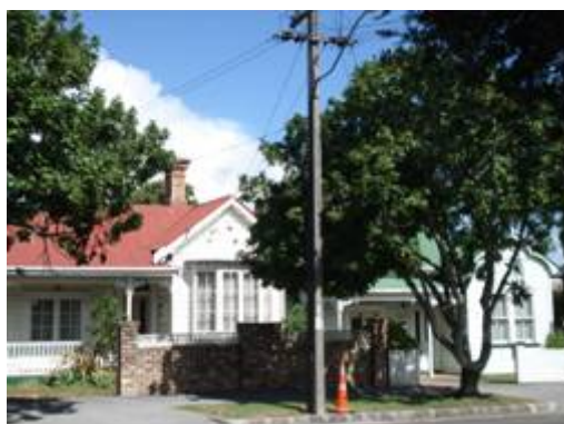
Figure 3.1 Example of an Auckland villa built in the 1900s
