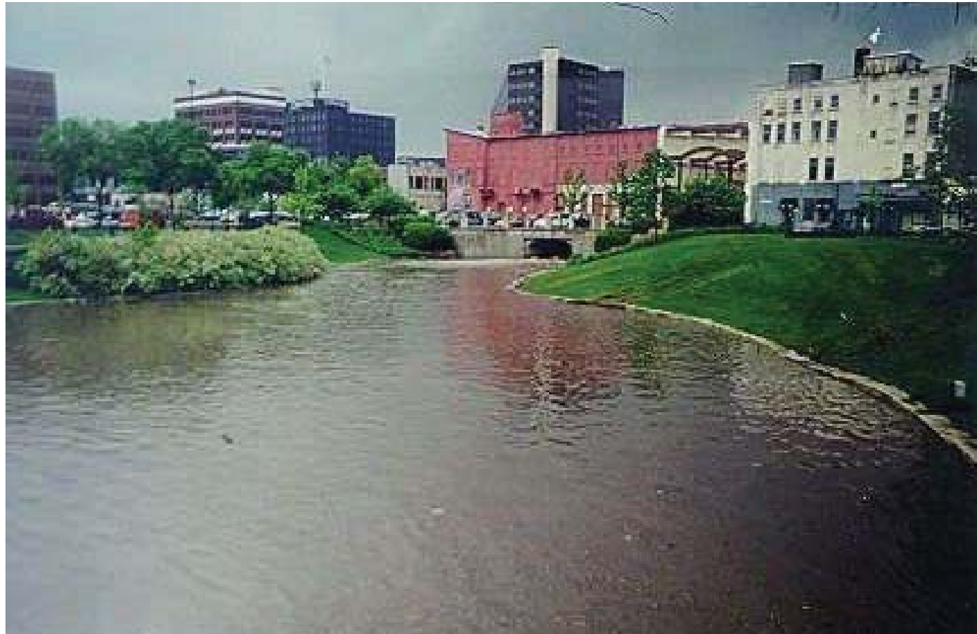
Daylighted river and associated public open space in downtown Kalamazoo, Michigan Courtesy of the Downtown Development Authority, Kalamazoo, Michigan
