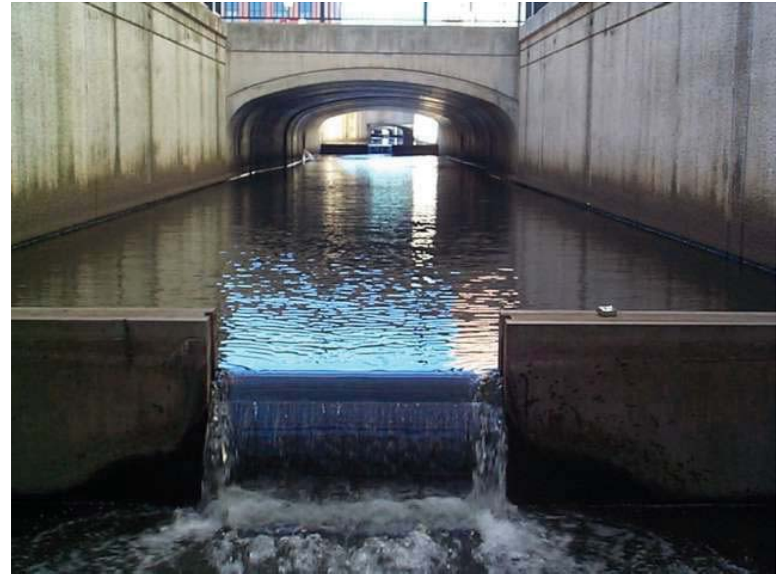
This daylighted stream in Kalamazoo, Michigan is channelised for much of its length, but has acted as a catalyst for many stormwater management initiatives in the catchment to enhance water quality
