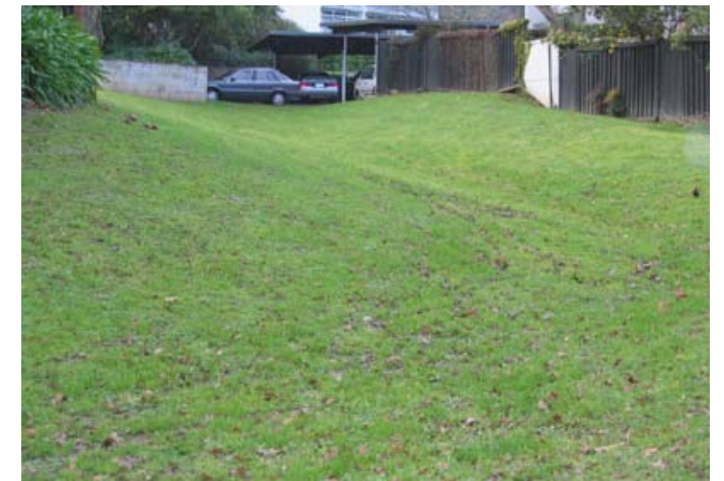
Overland flow path through Freemans Park housing estate as a potential site for daylighting
